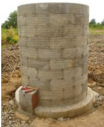
Figure 11 - ten layers of bricks completed (2m high x 1.57m diameter)
