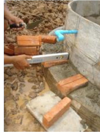
Figure 9 – Starring the outlet tap box
