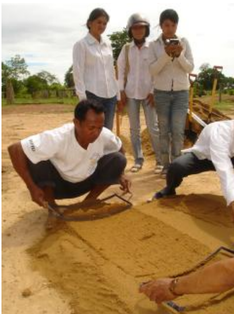
Figure 1 - Preparing for making the cement brick segments (3:1 sand to cement ratio)
