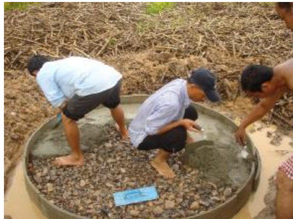
Figure 6 - Adding first cement layer to the rock infill
