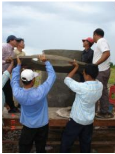
Figure 14 - Fitting the top covers
