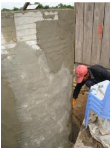
Figure 15 - Applying cement render to the outside of the tank
