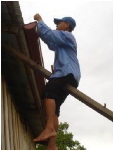
Figure 16 - Fitting the gutter to the roof
