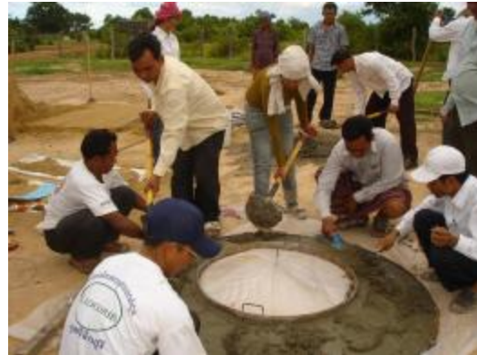
Figure 4 - Adding the cement to the top cover mold
