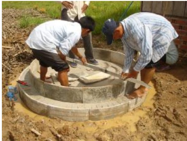
Figure 8 – Checking level of first layer of segments
