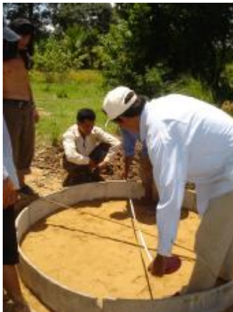
Figure 5 – Checking roundness of 12 bricks on base
