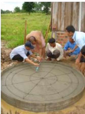
Figure 7 - Fitting wire frame and drain pipe prior to top cement layer
